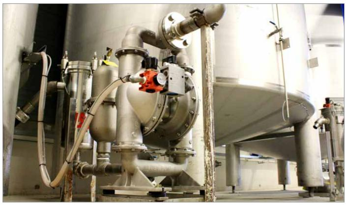
Correct diaphragm material selection for each application is critical to assure safe and efficient AODD pump operations.
