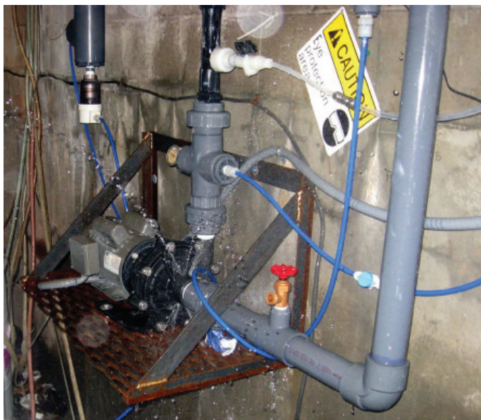
A mag drive pump caused a fluid rupture in a hazardous chemical application, putting workers at great risk.
