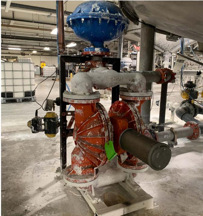
After seeing how Wilden® Chem-Fuse IPDs can improve service life and pump performance, Dunn-Edwards will begin standardizing the use of Chem-Fuse diaphragms on all of the 3" Wilden AODD Pump models in use at its Phoenix, AZ, manufacturing plant.
