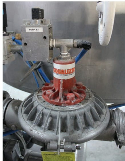
Havo employs a total of 25 Wilden pumps in its production operation and all are equipped with Wilden Equalizer SD Series Surge Dampeners. This optional accessory minimizes unwanted pressure fluctuations during liquid-transfer applications
