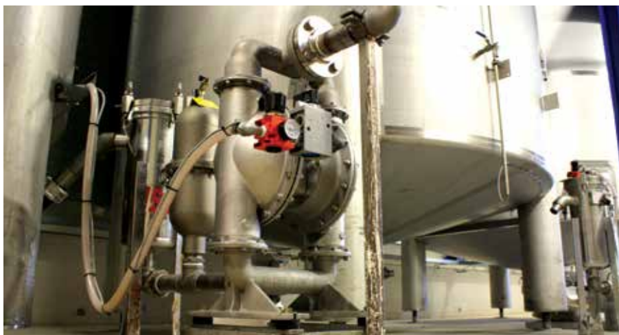
Image 2. A stainless steel AODD pump in a glue and adhesive manufacturing facility in the Netherlands
