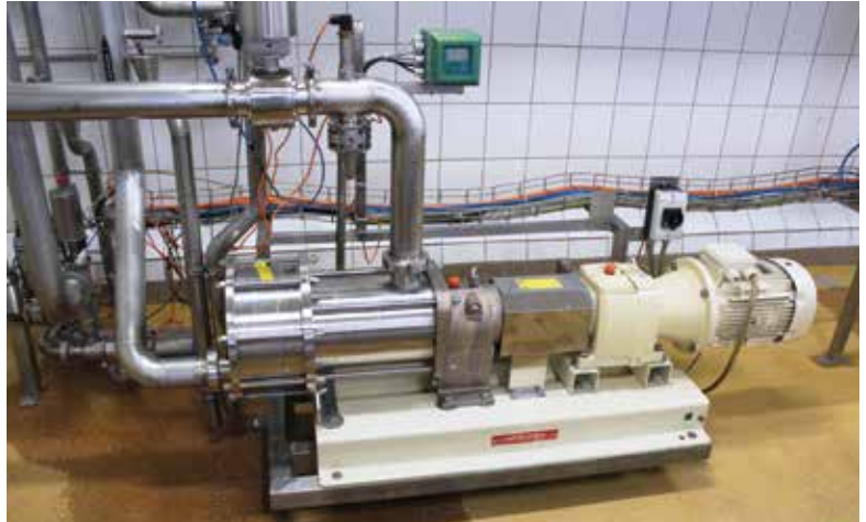
Image 3. An eccentric disc pump moving carbonated-beverages at a bottling plant in Hungary
