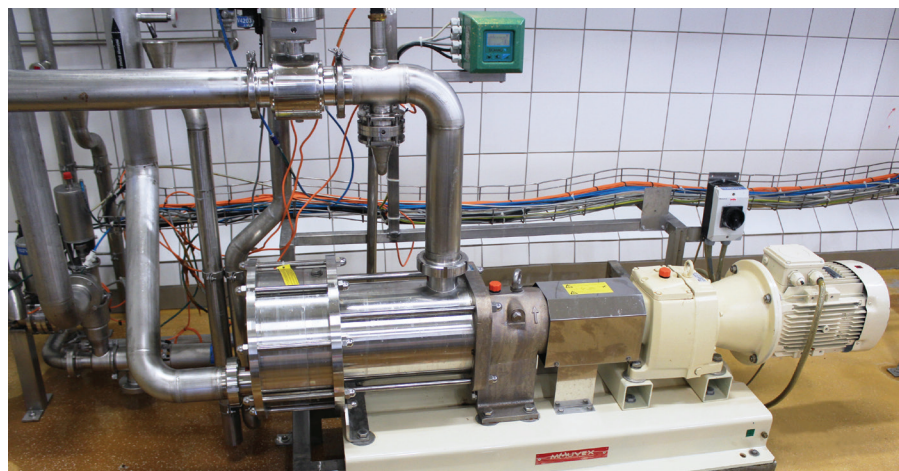
A Mouvex SLS Series Eccentric Disc pump being utilized for the transfer of carbonated-beverage bases by the Coca-Cola Hellenic Bottling Company in Dunaharaszti, Hungary.
