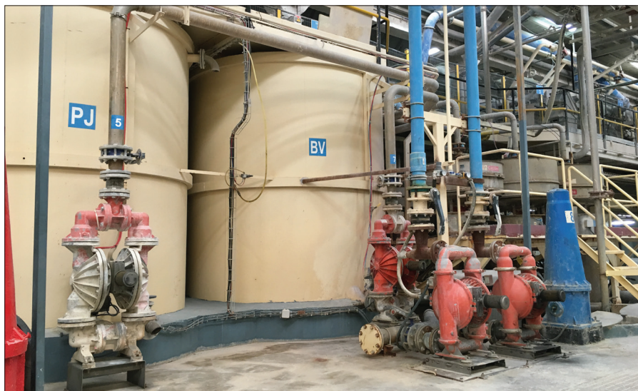
Wilden Original™ Series Air-Operated Double-Diaphragm (AODD) pumps in operation at a ceramic plant in Spain
