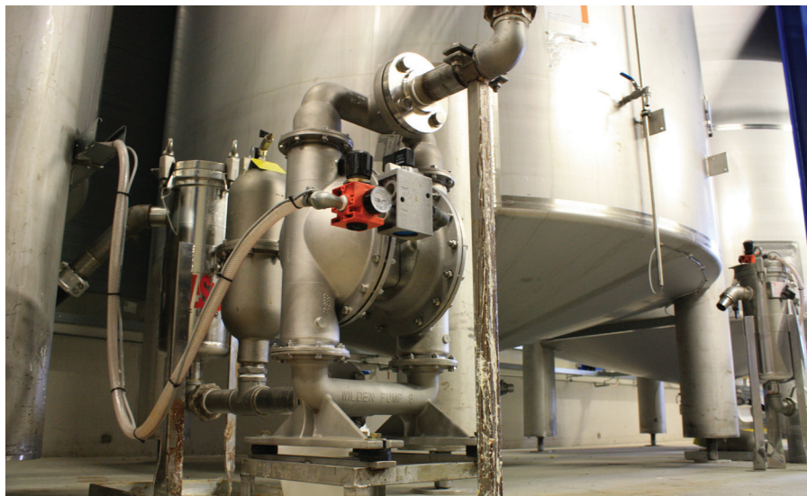
A stainless-steel Wilden Advanced™ PX Series AODD pump in use at the SABA B.V. glue- and adhesive-manufacturing facility in The Netherlands.
