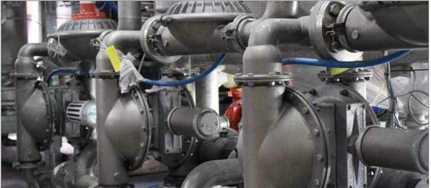
Wilden® Original™ and Advanced™ AODD pumps are the perfect solution for Havo thanks to their ability to handle high-viscosity liquids. Additionally, Wilden pumps feature a redesigned liquid path that reduces internal friction for maximized flow rates and pumping efficiency.
