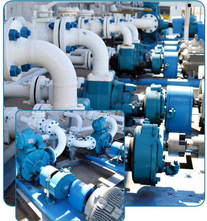
With their ability to produce an extremely accurate flow at lower volumes, Blackmer MLX and GX Sliding Vane Pumps provide low-volume blending of additives, ethanol and biodiesel.
