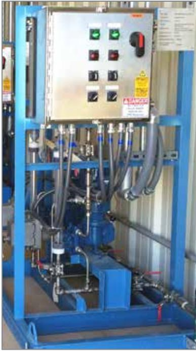
Hydraulically actuated diaphragm metering pumps are a leading technology of choice for wastewater-treatment plants because they can handle the harshest chemicals, can pump against higher pressures, offer highly repeatable dosing accuracy and have been designed for 20 year of service.
