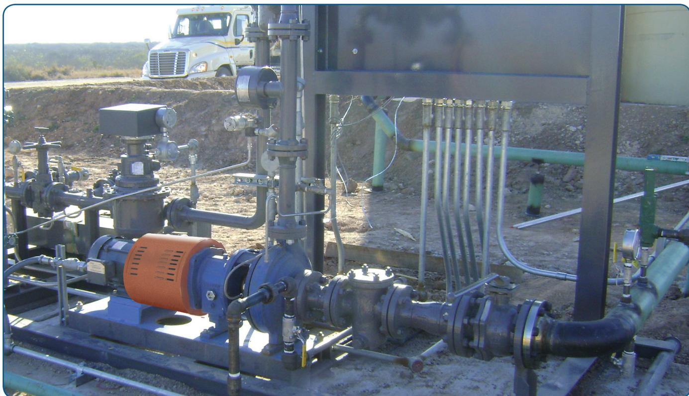
A new Griswold 811 Series installed in a Lease Asset Custody Transfer (LACT) unit located in the Eagle Ford play in Texas. A LACT unit automatically measures, samples and transfers the oil from a lease location in the oilfield into a pipeline.
