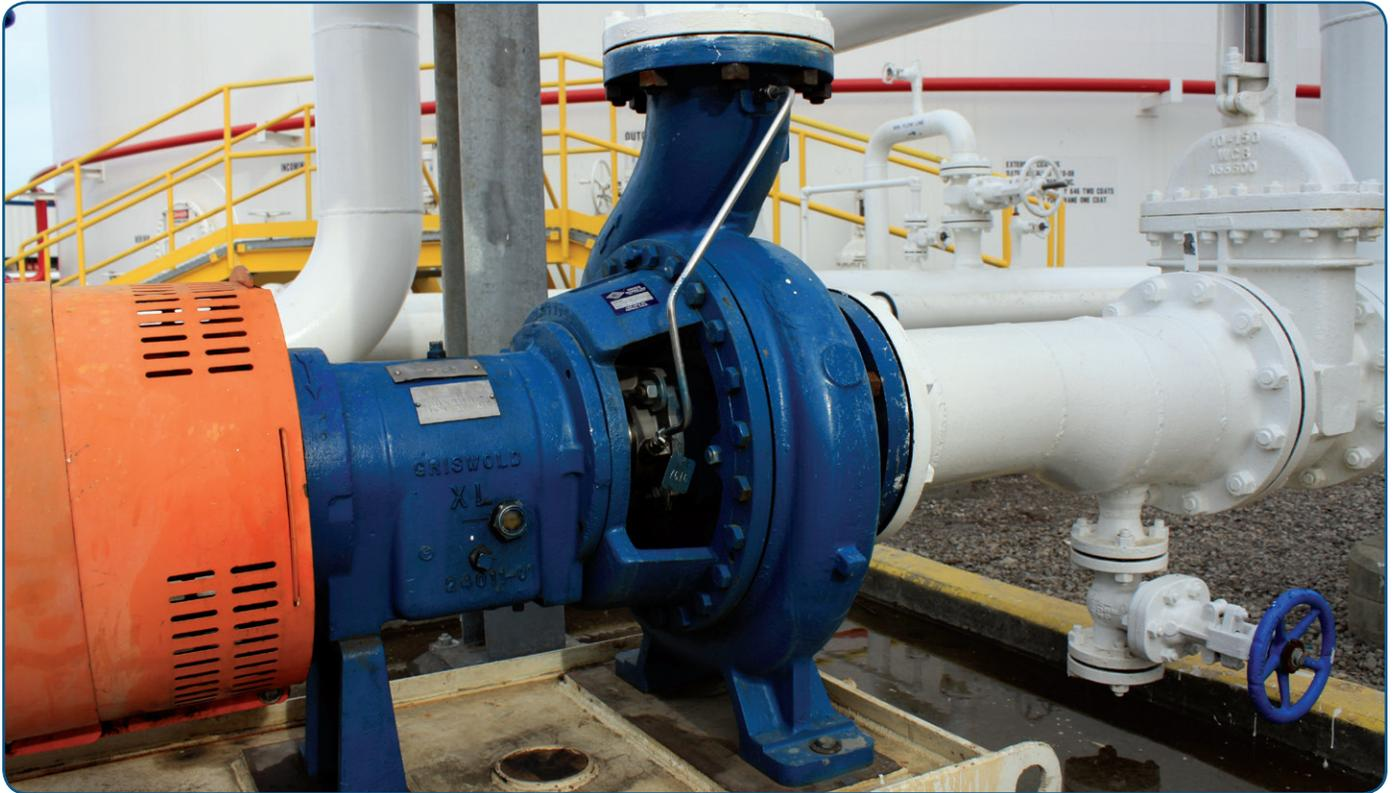
811 ANSI Centrifugal Pumps from Griswold™ Pump Company offer a method of manufacture that ensures that the “speed to market” requirements of oil and natural gas producers and refiners are satisfied.
