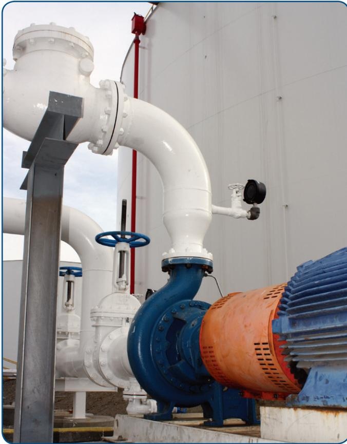
Griswold™ 811 ANSI Centrifugal Pumps possess the operational capabilities necessary to meet the demands of high-volume/high-flow liquid-transfer activities that are prevalent at refineries.
