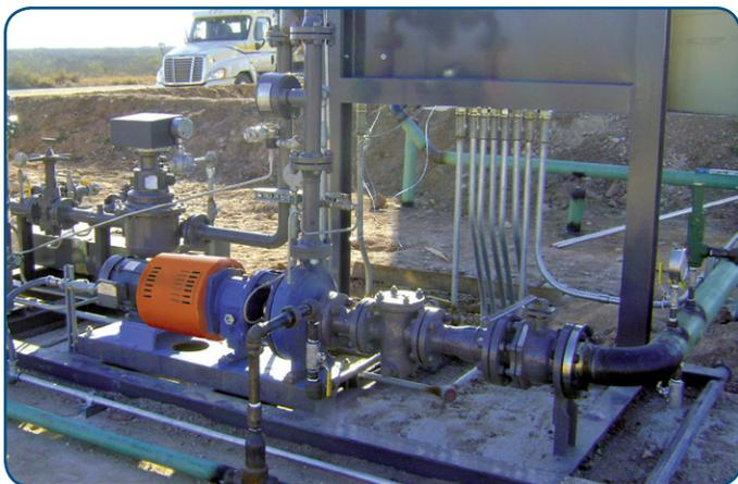
A new Griswold™ 811 Series pump installed in a Lease Asset Custody Transfer (LACT) unit located in the Eagle Ford play in Texas. A LACT unit automatically measures, samples and transfers the oil from a lease location in the oilfield into a pipeline.
