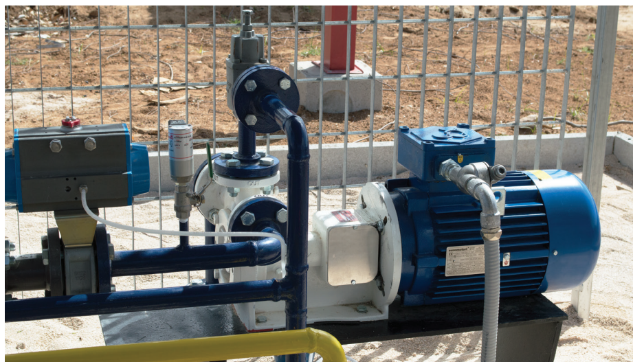
Ebsray® The RC40 pump will easily, reliably and economically produce differential pressures up to 14 bar (200 psi) with flow rates up to 200 l/min (52.8 gpm)
