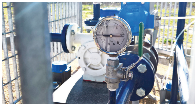
When fuelling begins, the Ebsray RC40 Series Regenerative Turbine Pump can create 21 bar (305 psi) of pressure
