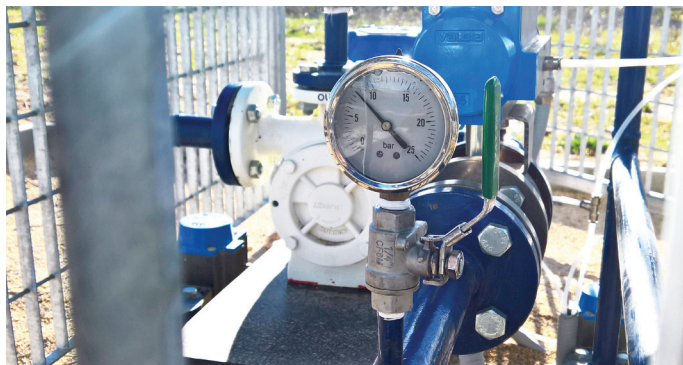
At rest, the Autogas storage tank at AmeGas' site in Sabaudia has a pressure of 8 bar (116 psi)
