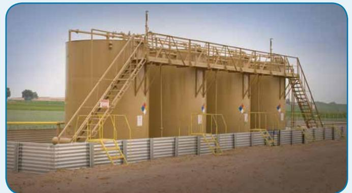
When crude oil is gathered and stored in a tank battery the chance for vapor escaping is very high. Vapor-recovery systems that feature Blackmer Oil-Free Reciprocating Gas Compressors can capture these vapors providing increased safety and additional revenue for the producers.
