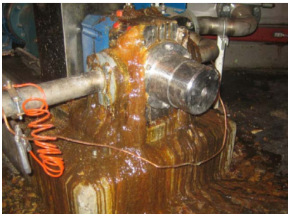
These are a few examples of what can go wrong when pump styles with inadequate product-sealing capabilities are used in resin-handling applications.
