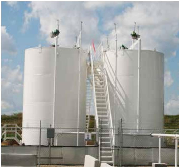
*In-the-field storage tanks are used to house raw crude oil and natural gas before it can be transported for refinement. Operators must control the amount of potentially harmful vapors that are released to the atmosphere from the tanks and are turning to vapor-recovery units as a solution.*
