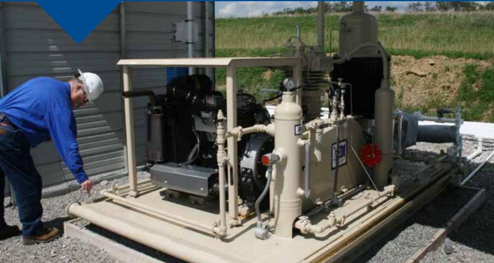
*The use of vapor-recovery units in the oilfield is on the rise, for both economic and environmental reasons. Blackmer® Oil-Free Reciprocating Gas Compressors are vital components in many of these installations.*
