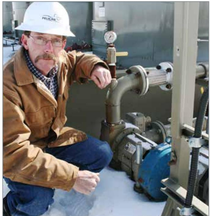
As part of his responsibilities, Tom Roberts, Field Supervisor for Pelican Gathering Systems, monitors the Pelican pipeline system, which utilizes pumps to introduce the oil and natural gas into the pipeline at the wellhead, transfer it through a series of switching locations along the pipeline and then deliver it to the storage tanks.
