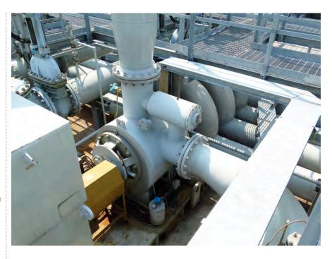
fluid is shifted and steadily and constantly conveyed to the discharge port of the pump, which creates a volumetrically consistent flow rate regardless of the pumping pressure.
