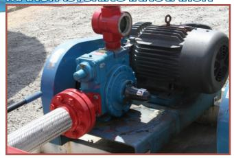
At its dual-transport loading island, Rockville Propane Terminal utilizes LGL4 series sliding vane pumps from Blackmer®. Designed for maximum performance and reliability, LGL4 pumps incorporate a wide variety of design features that help eliminate maintenance and downtime.
