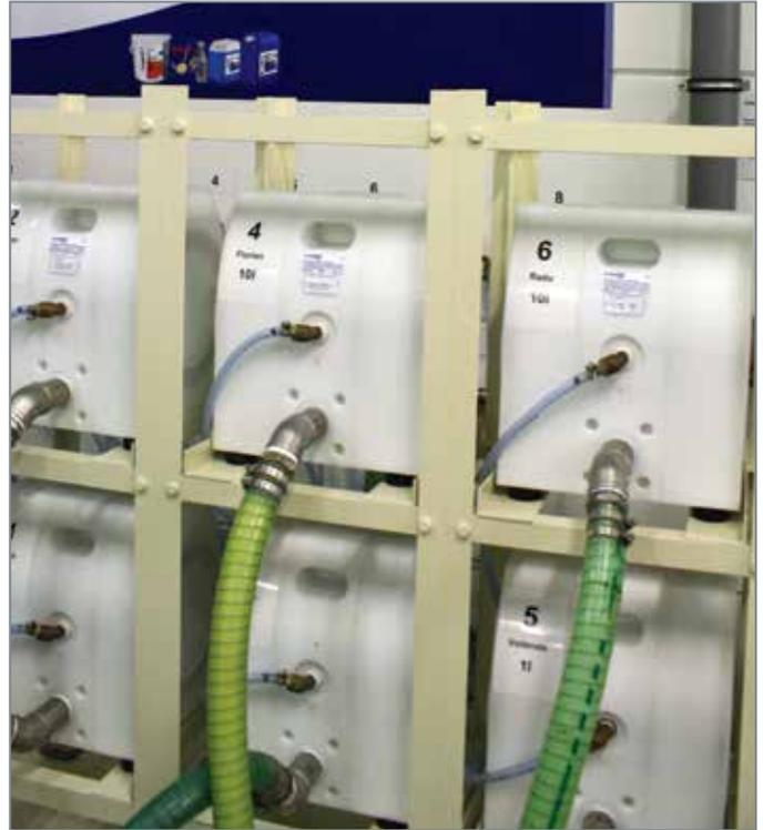
Almatec® E40 Series AODD Pumps are the perfect pumping solution for Langguth Chemie because they are able to meet the demands of stop/start continuous-duty pumping applications while consuming less air and generating less noise.
