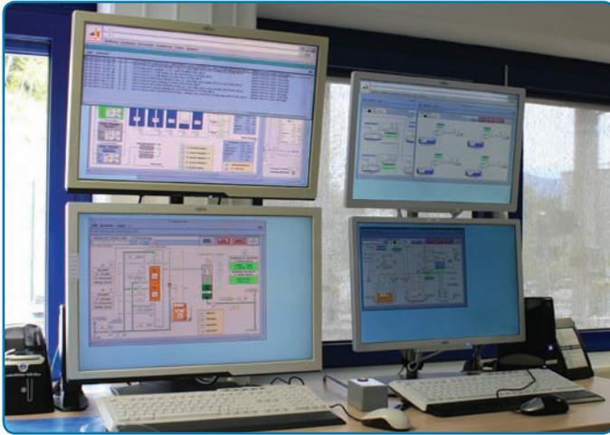
Roche Diagnostics' used-solvent storage tanks are monitored from a dedicated on-site computer room that gives the operator real-time information regarding liquid levels and potential alarm conditions.
