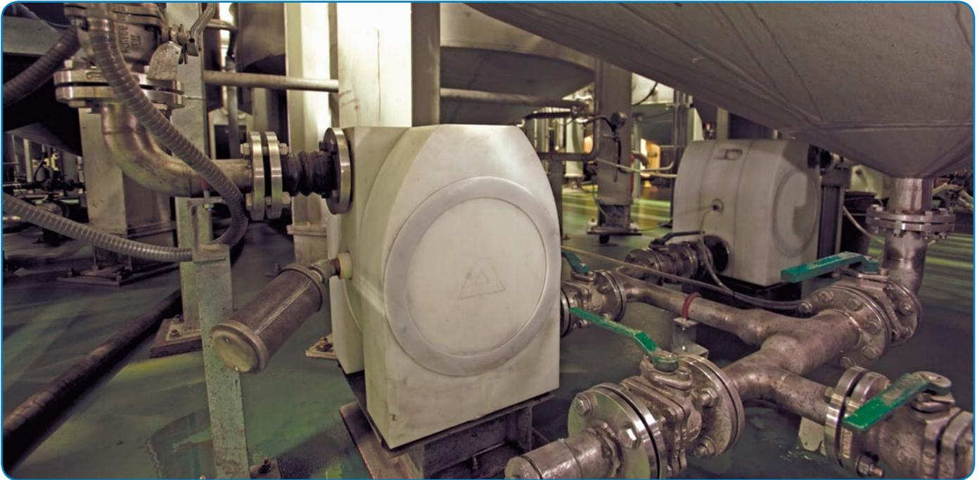
Almatec E-Series pumps installed at one of CRS Reprocessing Services' newest slurry reprocessing facilities in Korea. Almatec E-Series pumps are ideal for harsh slurry applications thanks to a solid body design constructed with PE material, which has an abrasion resistance that is 7 times higher than that of polypropylene and 1.6 times higher than steel.
