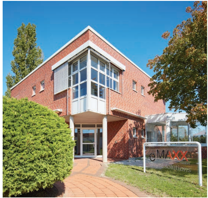
eMAXX conducts business for the semiconductor and other industries at its state-of-the-art production facility in Merbtiz/Dresden, Germany.
