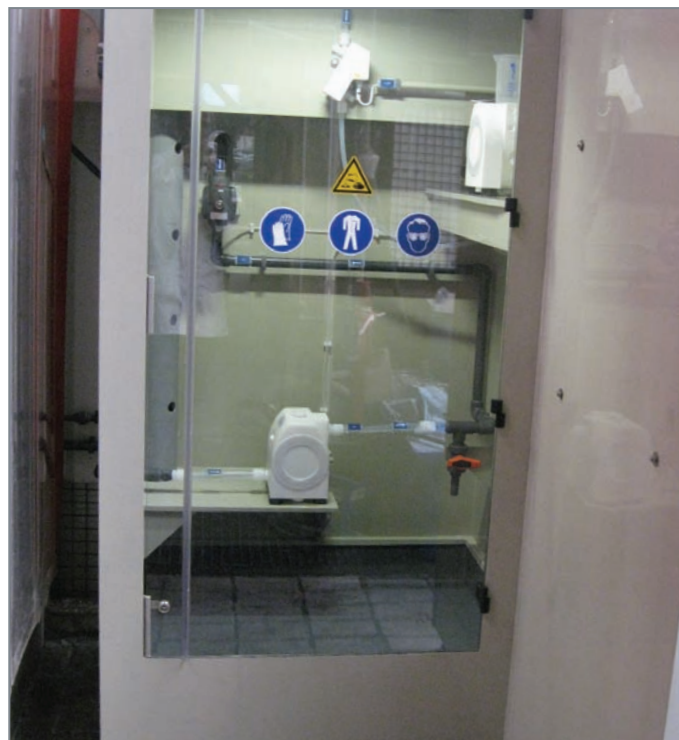
Many high-purity chemicals can cause compatibility concerns when used with certain types of pumps. Almatec® E-Series AODD Pumps can be constructed of plastic materials that are specifically compatible with the chemicals that are being handled, which eliminates cross-contamination and leak fears.
