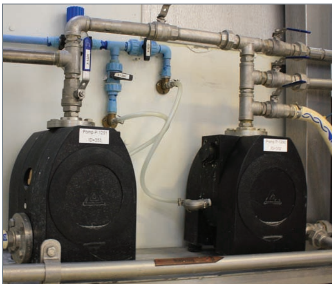
The plastic solid-body construction of Almatec® E-Series AODD Pumps eliminates the small crevices or cavities that can be found in injection-molded models. It is in these crevices that liquids can accumulate and leak paths can be created.
