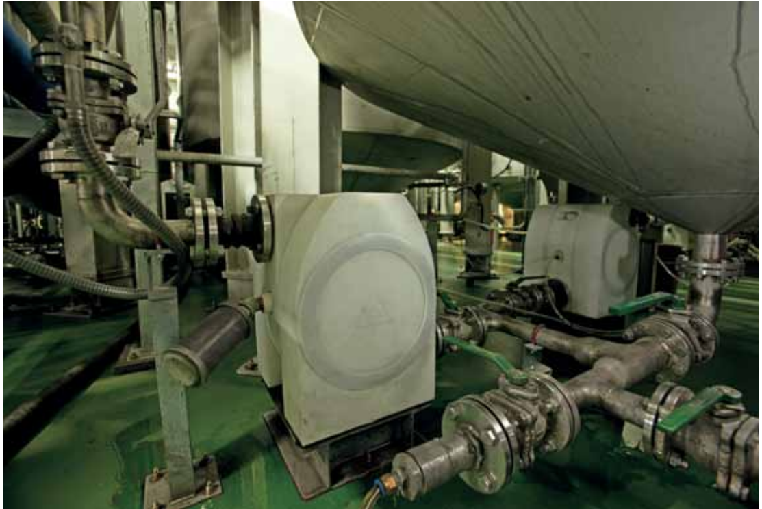
AODD pumps are ideal for harsh slurry applications thanks to a solid body design constructed with PE material, which has an abrasion resistance that is seven times higher than that of polypropylene and 1.6 times higher than steel.
