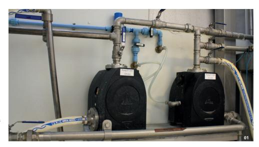
rosive, the pumping equipment used to transfer them is prone to chemical attack if the materials of construction are not compatible with the acid, caustic or solvent. Another area to focus on is the actual design features of the pump. For example, if the design incorporates mechanical seals or packing, they may be prone to leaking.
