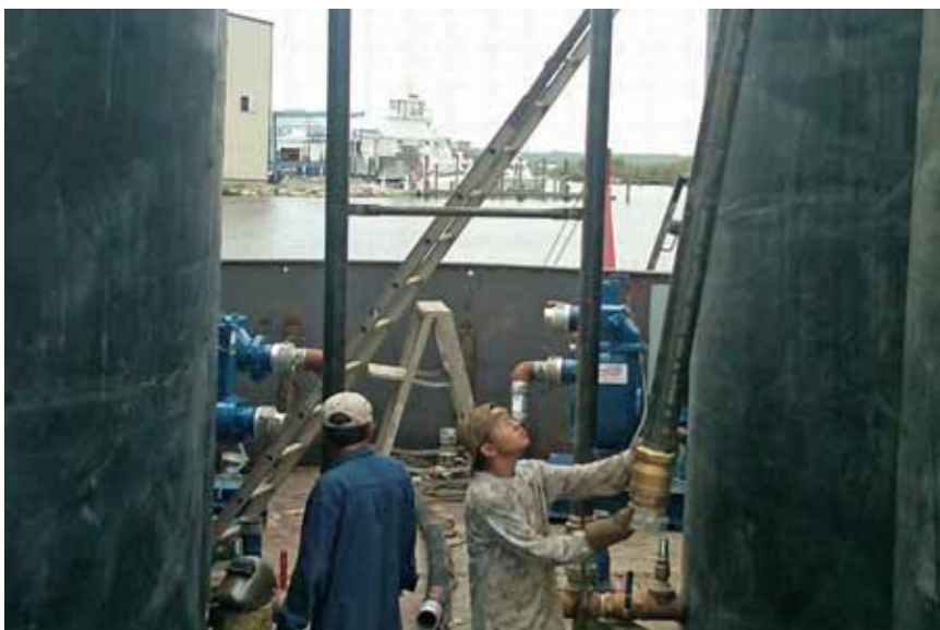
Workers installing Thompson pumps onto transfer barges.
