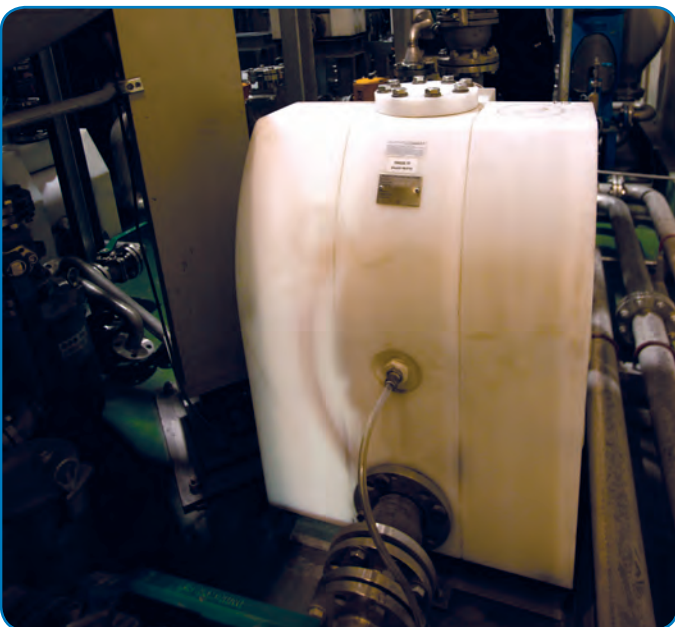
The solid body construction of Almatec's E-Series pumps provides a wide range of advantages to the end-user, such as increased pump safety due to an innovative ring-tightening structure.
