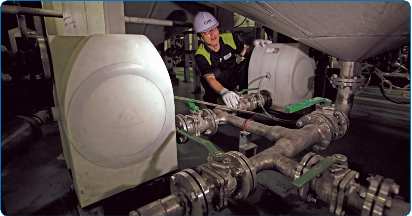
The housing on Almatec's E-Series solid body AODD pump is constructed in polyethylene (PE) and polytetrafluoroethylene (PTFE), which are both ideal for solar cell production. Almatec E-Series pumps are pictured here in a slurry application found in a plant owned by CRS Reprocessing Services.
