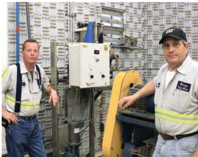
UPPER PHOTO: Operator Tim Mack, left, and Jay Berman, superintendent of the City of Marengo Wastewater Treatment Facility, use the dynaBLEND liquid-polymer activation and blending system from Fluid Dynamics, a division of Neptune Chemical Pump Co. RIGHT PHOTO: The processed biosolids material is eventually used as fertilizer.
