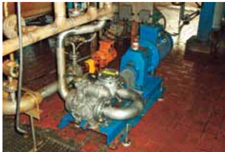
Above: Sealless sliding vane pump transferring polymer dispersions
