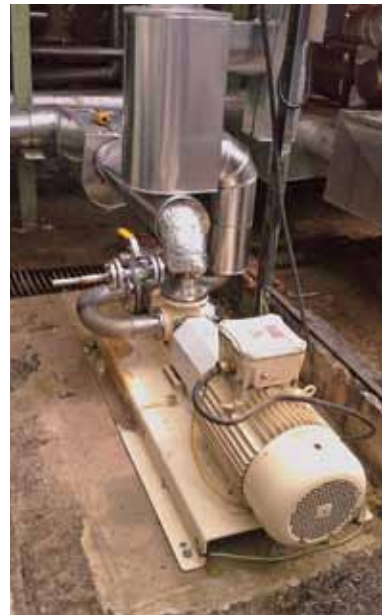
Above: Sealless sliding vane pump transferring polymer dispersions
